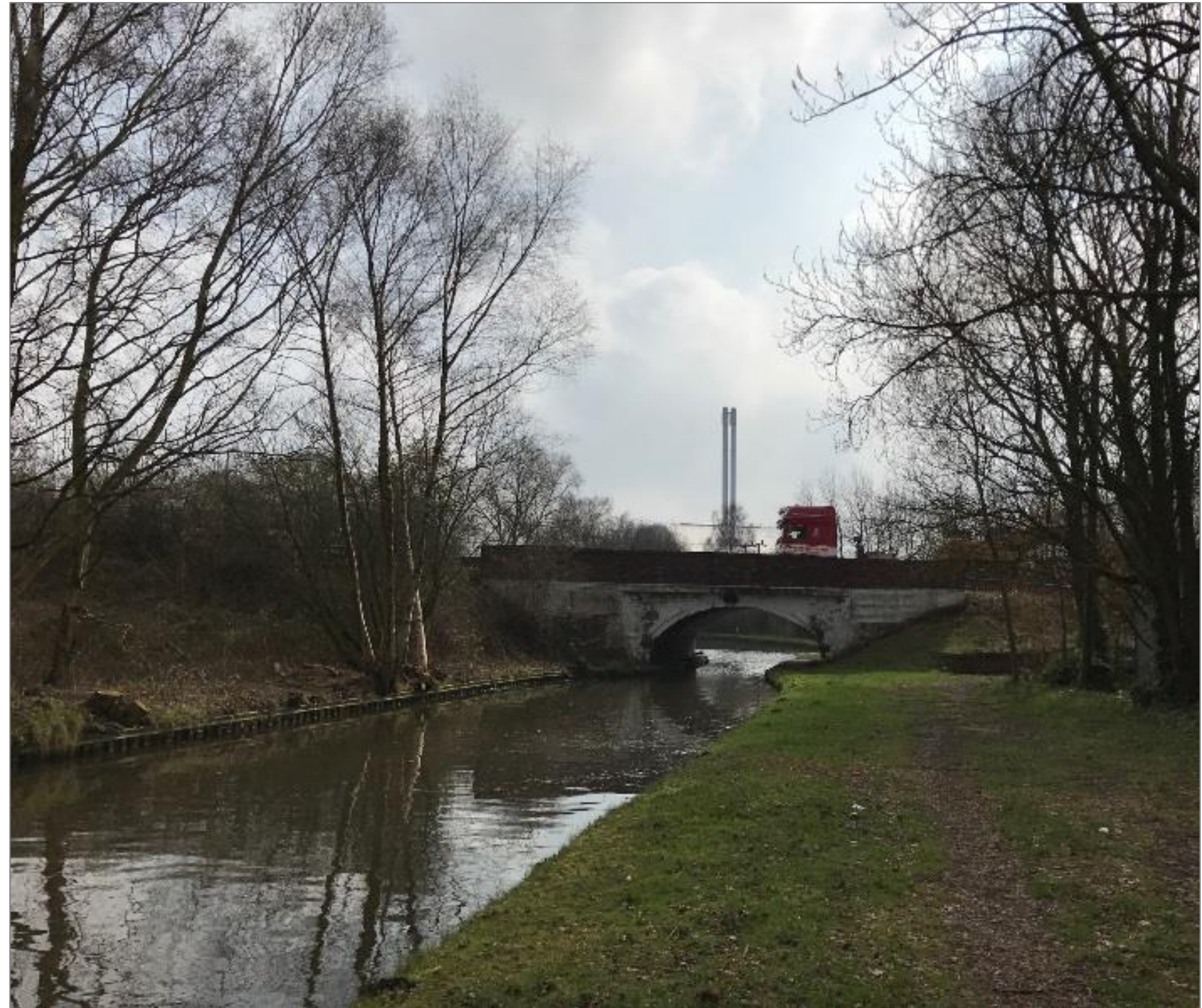
Figure 10: View looking south along the Canal towards the Veolia Energy Facility (July 2017)
