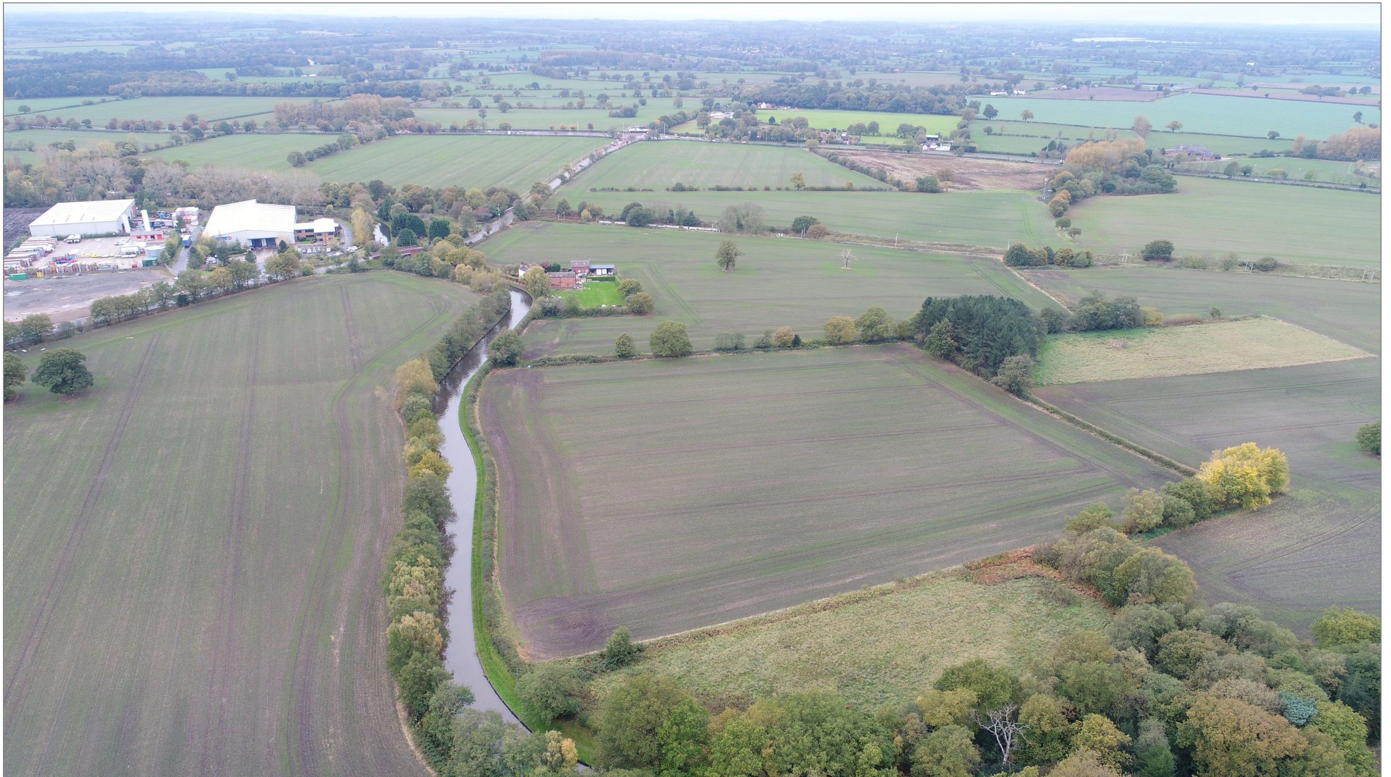
Figure 4: Aerial image of the Staffordshire and Worcestershire Canal running through the Site
