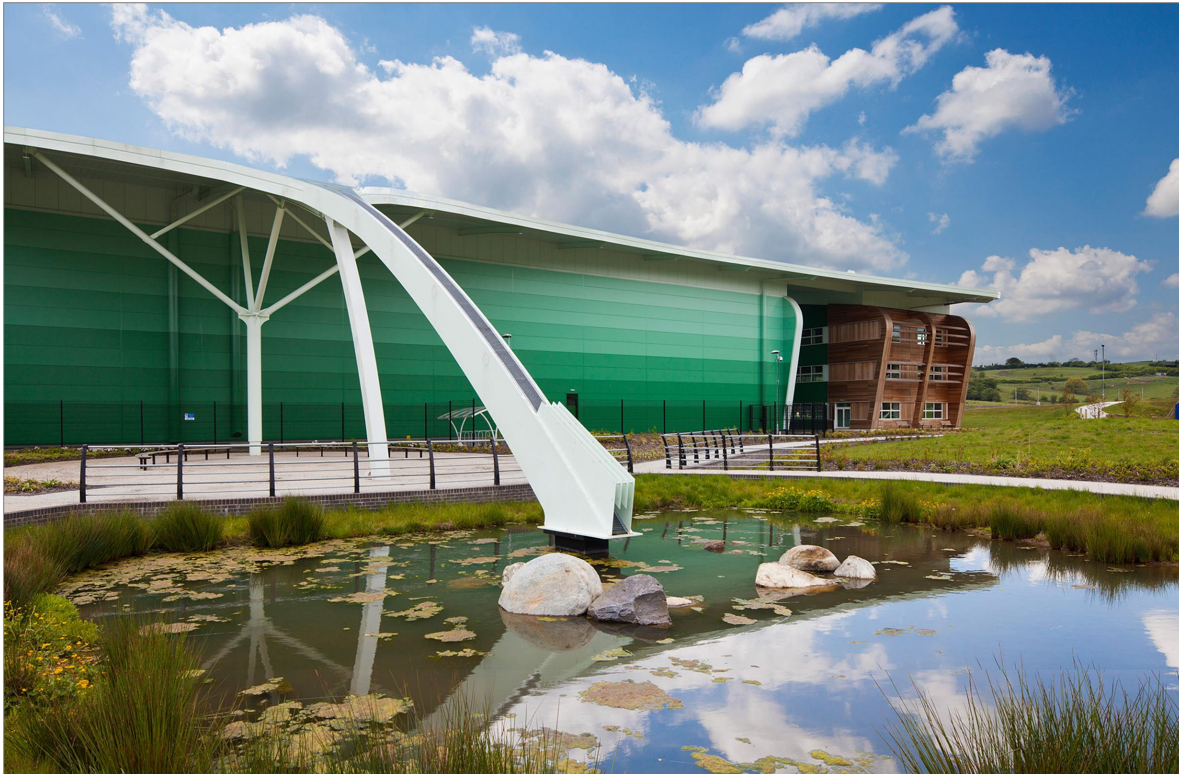
Figure 68: A high quality distribution building in Chatterley Valley, Stoke designed with consideration to the surrounding landscape
