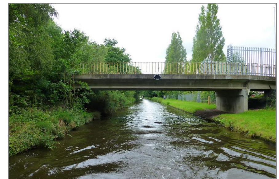
Figure 75: Redundant Access Bridge over the Canal
